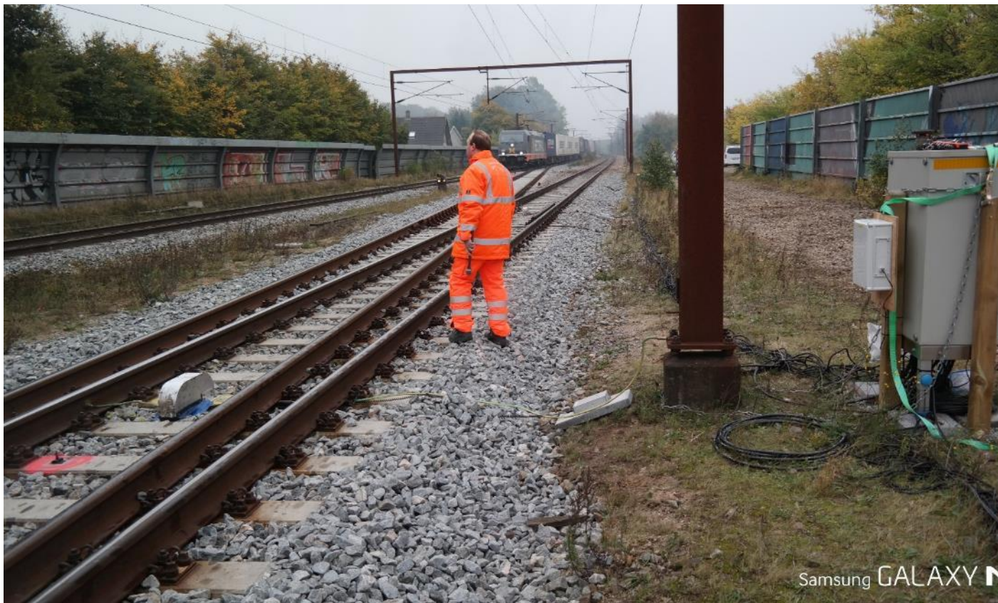
Figure C1 Tommerup test site overview - switch on left, cabinet with installed gateway on right
