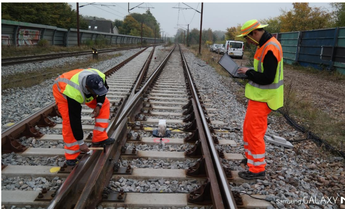
Figure C6 Setting sensor threshold for incoming trains
