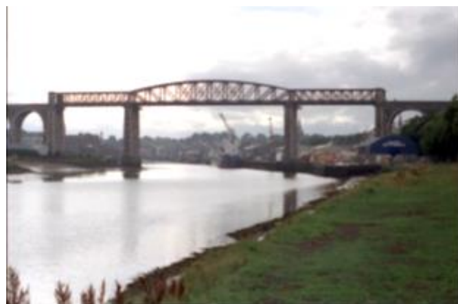
Boyne Viaduct Ireland which is one of the project case studies
